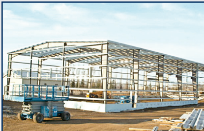
Steel-frame Welding Shop
