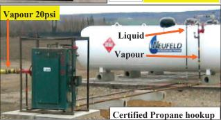
6.4 mbtu N/G Burners | Oil collects in bottom of tank so both lines draw from the top
